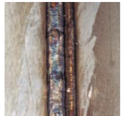
Figure 5: Vertical weld between corrugated tank walls; mechanised welded with OK Tubrod 14.27
